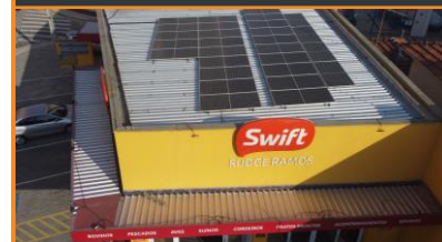
55. Rudge Ramos - 16,38 kWp
